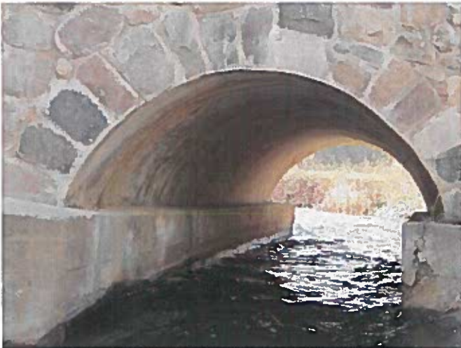
Document Name: 031.JPG Category: Other Span Number: Comments: Typical arch interior.
